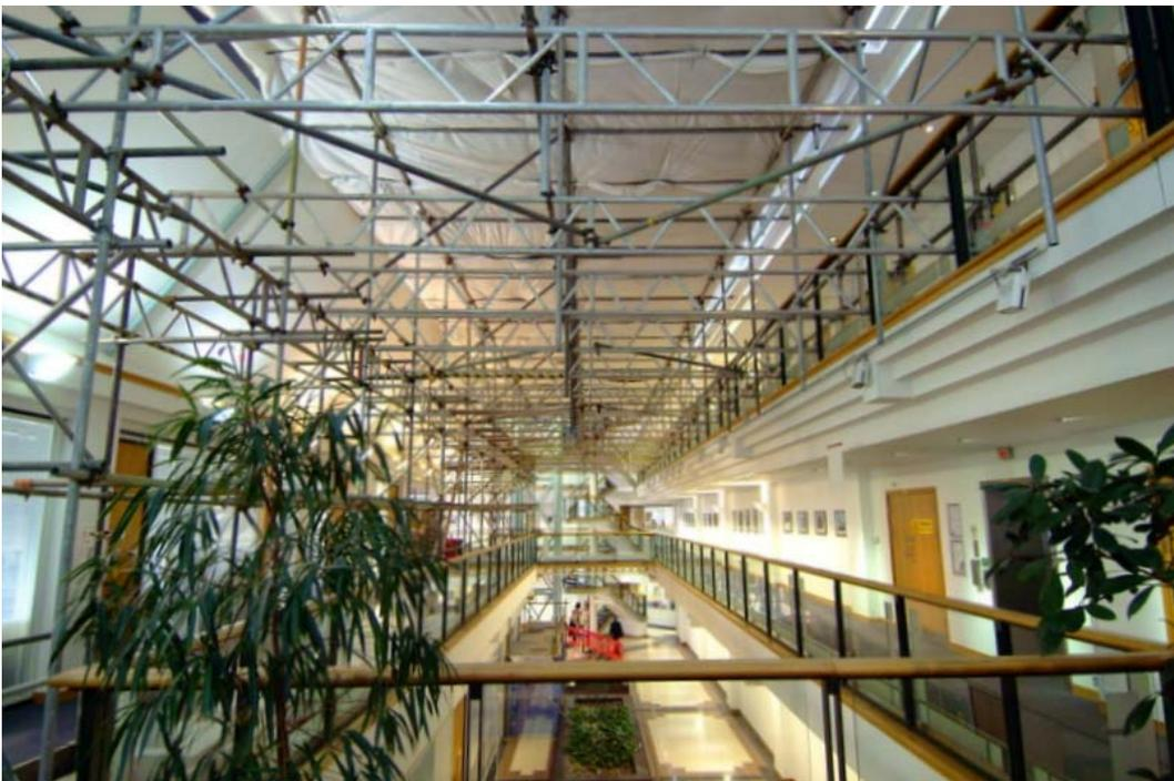
The existing glass was removed in batches, and the new glass installed in a rolling programme, to minimise Client disruption. Working in occupied areas involved very careful programming, and phased erection of access scaffolding both inside and outside the building.
