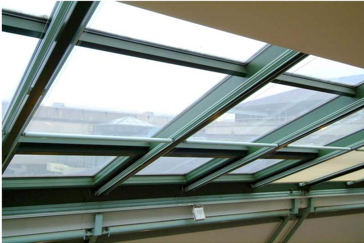
It was established that the original Shueco glazing system was 'upgradable' and could be retrofitted on the existing structural rafters using thicker, more energy efficient 31mm glass units, with new external pressure plates, thermal breaks, cover caps, etc. Approximately 777 bespoke glazing units, many to shaped angles, etc, had to be measured, manufactured, delivered, moved to the various locations, and fitted in position, over the 12 month contract period.
